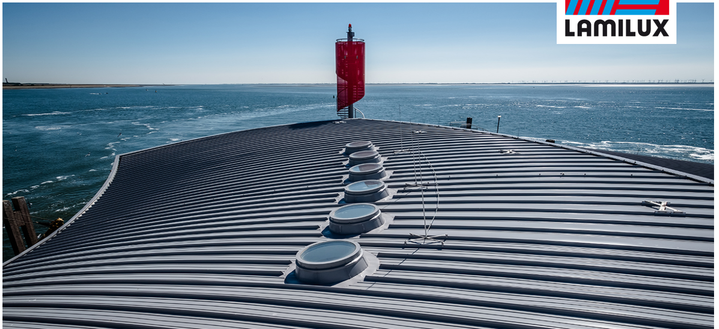
Harbour Terminal "Hafendüne", Norderney (Germany)
